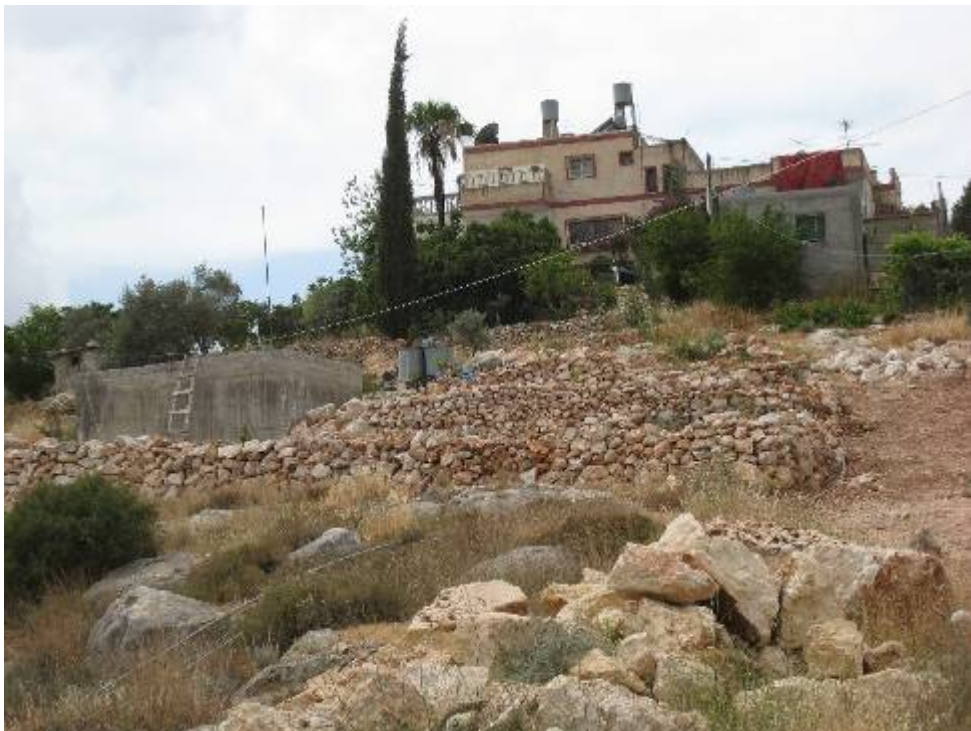
The house of Bassam Qdah in Shukba in the OPT, and the family's water cistern, which is threatened with demolition © AI
