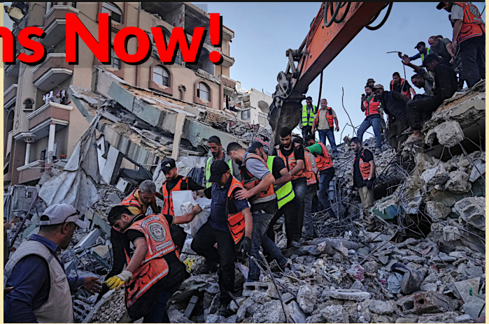
At least 21 people including 11 children died after a war-damaged residential building in Gaza City collapsed on 16 September, with dozens more feared trapped under layers of rubble. photo: Jihad Alshrafi/AP
